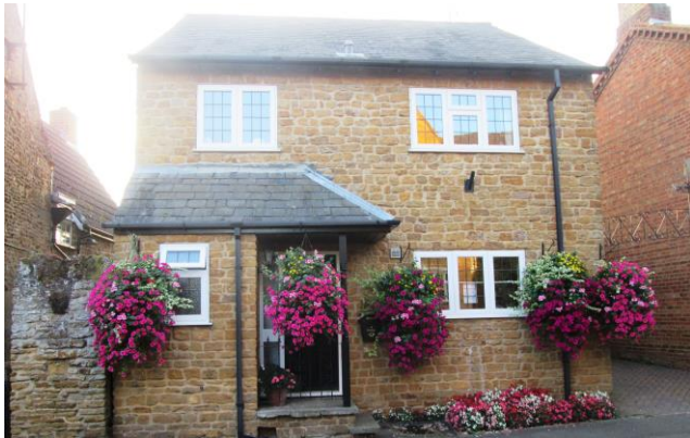
Example of infill development, High St
