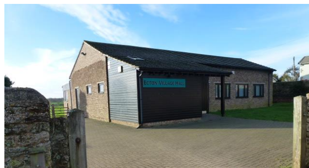
The village hall – a vital community facility
