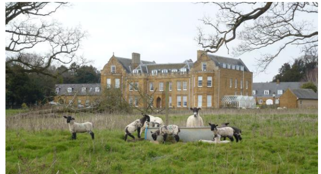
View of Ecton Hall from the Ecton to Earls Barton public footpath (TE1)
