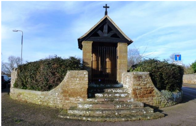
The war memorial. An example of a structure which is not listed but should be assessed for inclusion on a local list of heritage assets.
