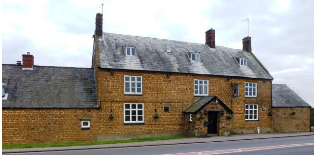
World's End, Northampton Rd - a Grade II Listed Building
